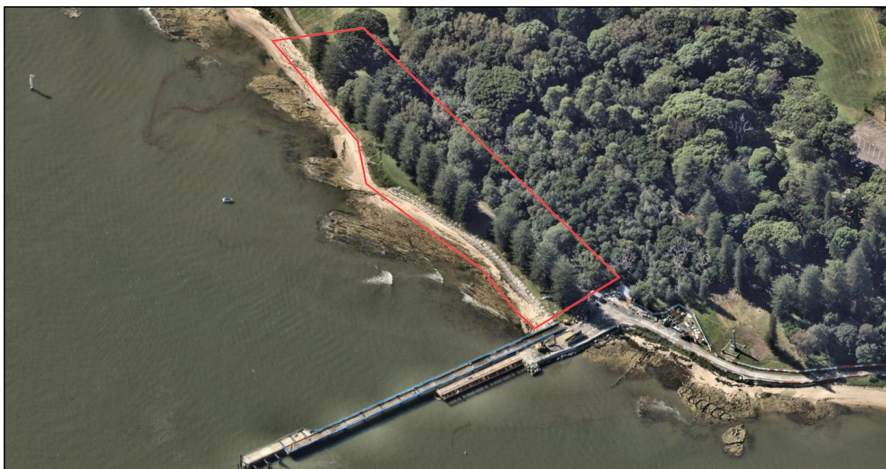
Figure 7: Oblique view of the area of proposed works, with existing sandbag wall and Kamay Ferry Wharf visible (under construction)
